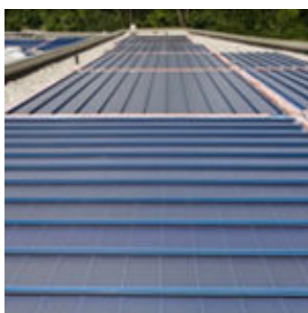
Figure 3: Flexible Photovoltaics on a U.S. Rooftop
