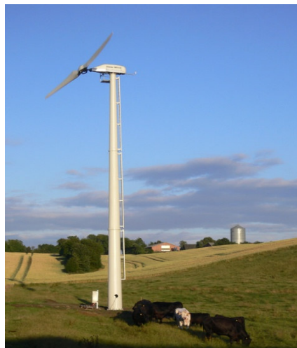
FIGURE 3: GAIA 11 KW WIND TURBINE INSTALLED AT A FARM.
